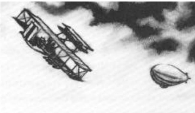
Later, the French also used the first air-launched rockets, again, against zeppelins. Nieuport biplanes were outfitted with racks for four rockets on each wing strut and their use against captive balloons was credited with forcing the Germans to discontinue use of this type of observation aircraft.
