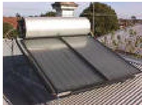
**Figure 12.1 Solar Flat plate collector**
